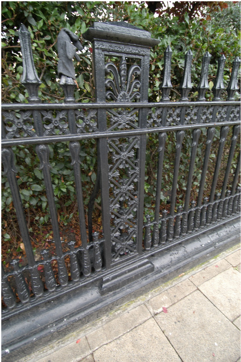
Photo no. 13 Flat front standard with backstay Listed Railings RL15 (part of EH list entry no. 1244298)
