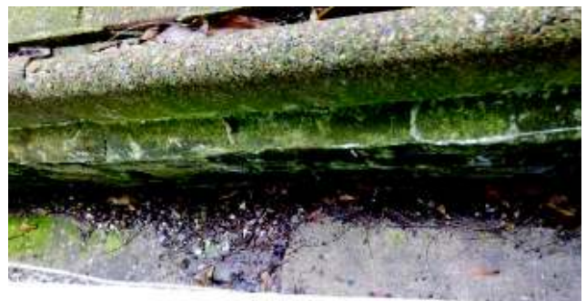
Fig 1.4 – Retaining wall to raised patio.
