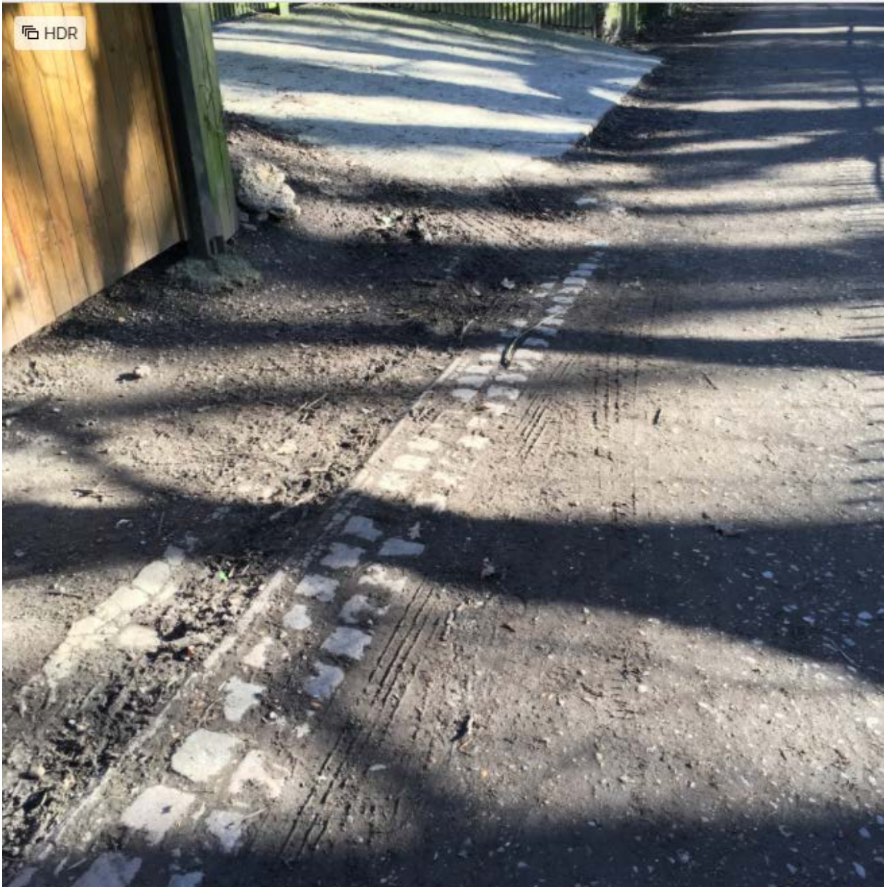
Image 8: Typical vehicle tyre rutting
