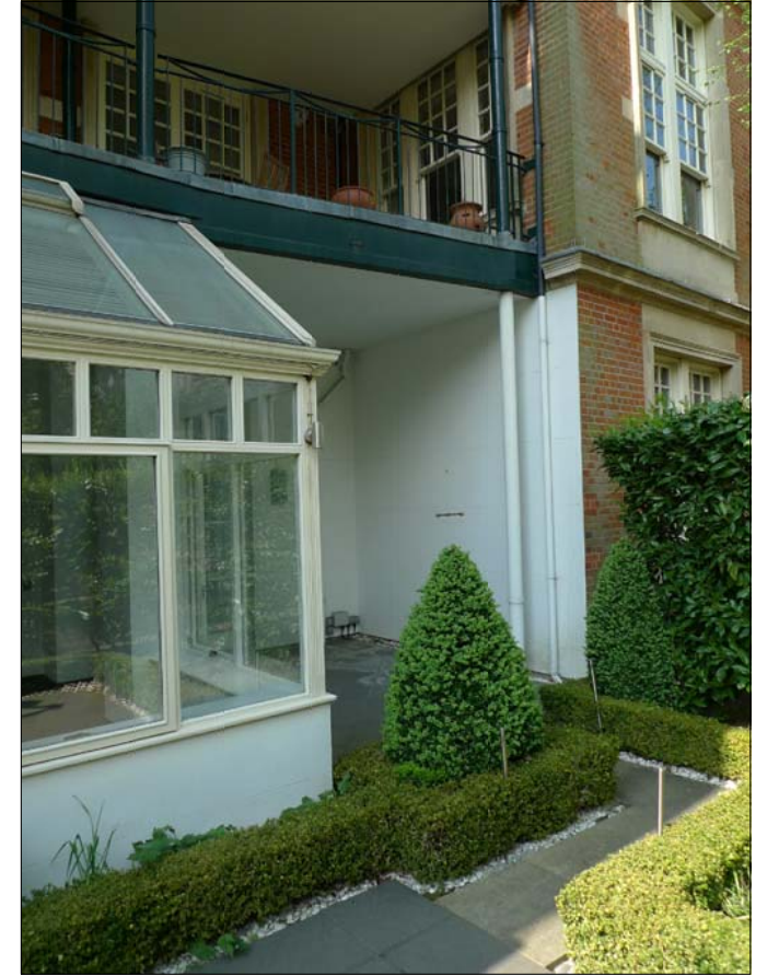
Existing glass extension, view towards North East
