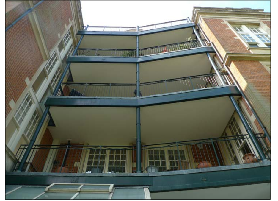
View onto the balconies above
