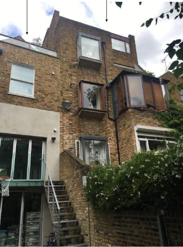
Image 2. Rear Elevation showing no. 5 King Henry's Rd.
