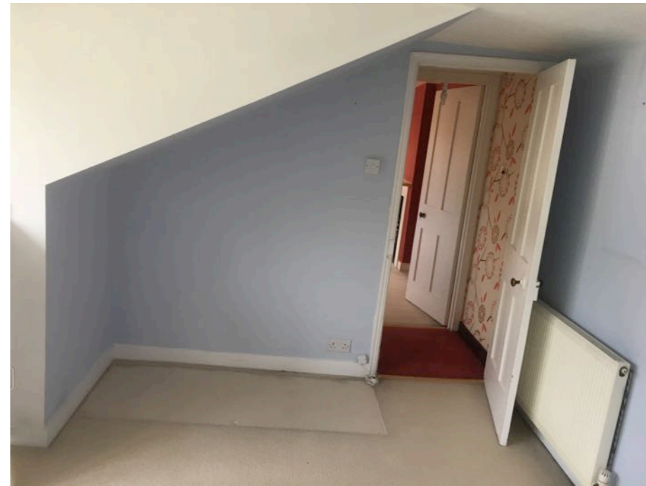
Existing Second Floor Bedroom Skirting
