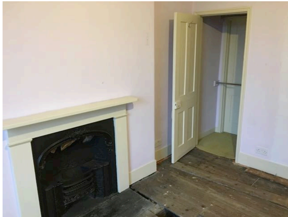
Existing First Floor Bedroom Skirting
