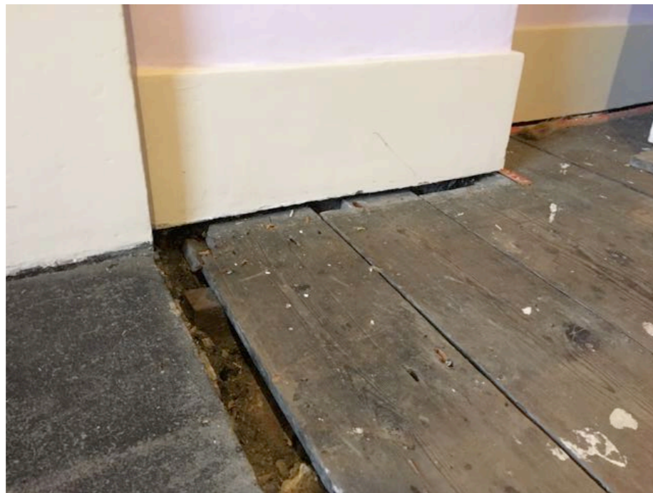
Existing First Floor Bedroom Skirting Detail
