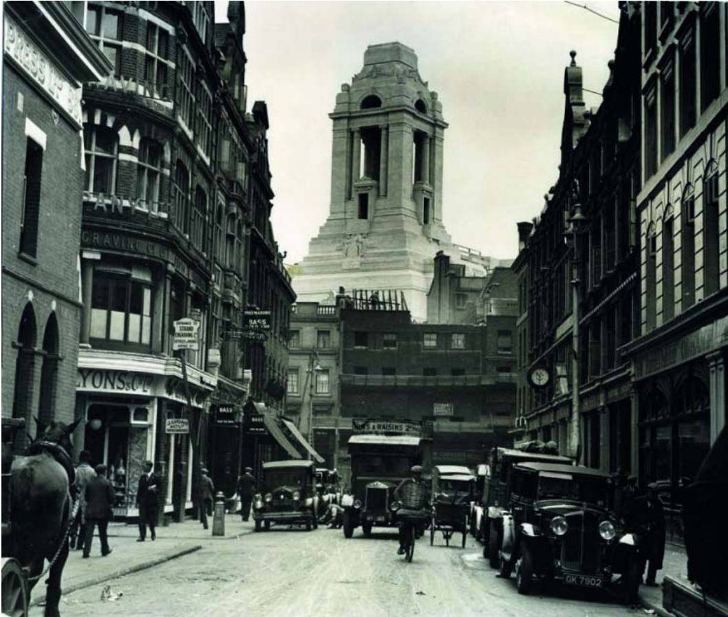
Figure 7: View over partially demolished buildings 1931 (©UGLE)
