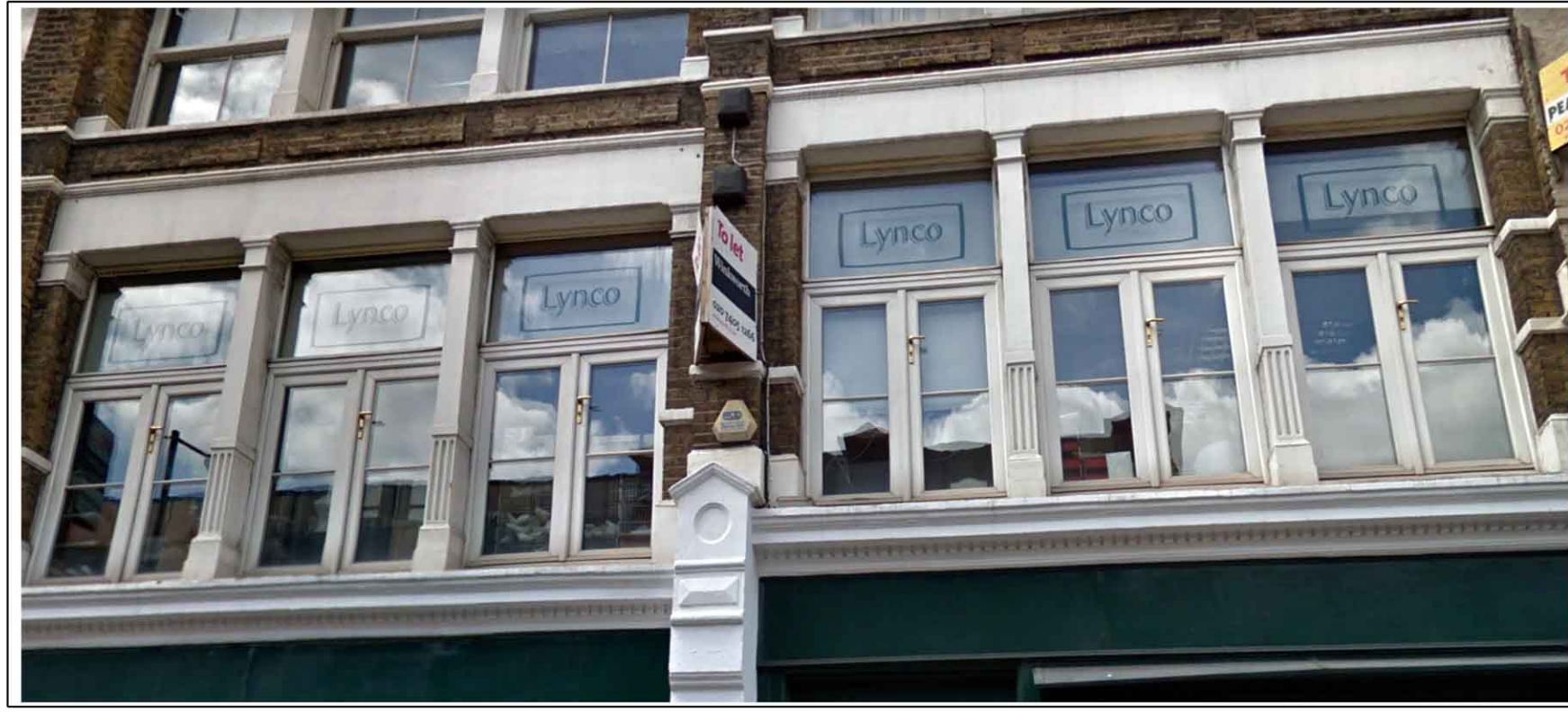
View of the upvc windows from the street
