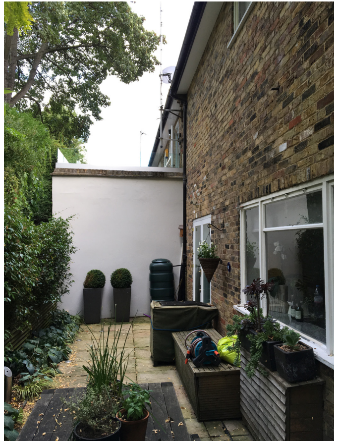
View C - Existing garden and rear elevation looking East
