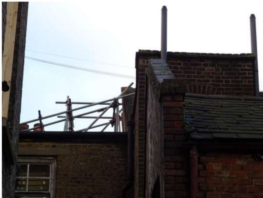
Figure 4.8.9 Gable End to No.26
