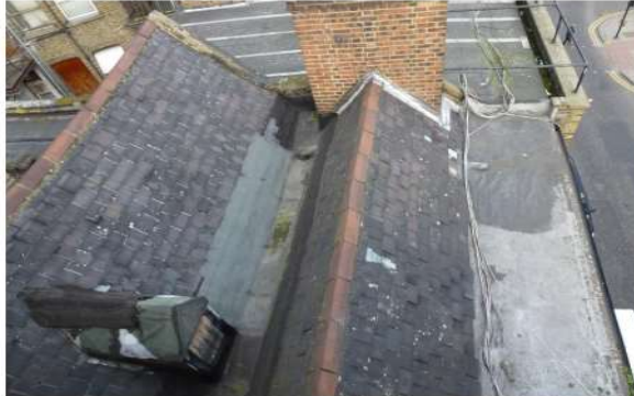
Figure 4.8.10 Valley in Roof to No. 26
