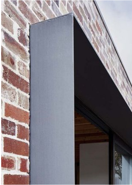
Projecting window cuff on first floor picture window and second floor window
