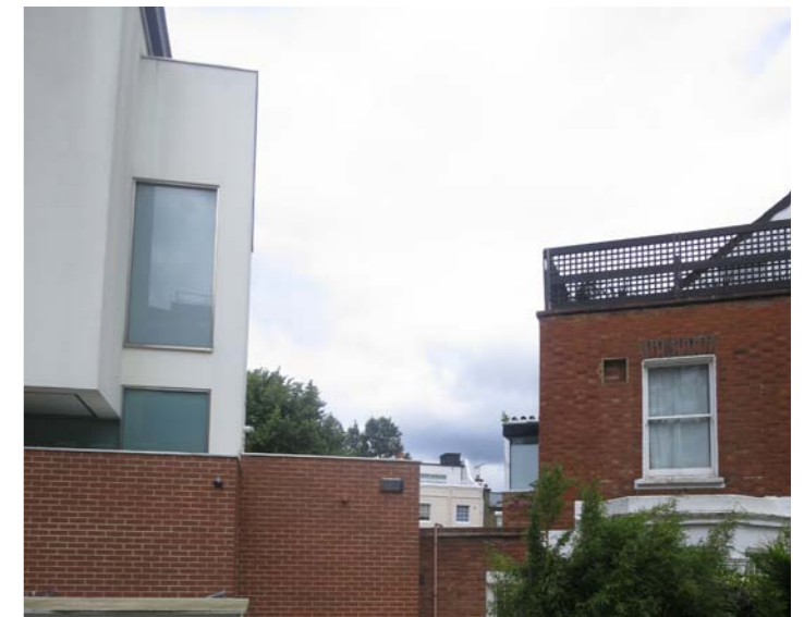
Gap between no. 35 Pilgrim's Lane and 49 Denning Road.
