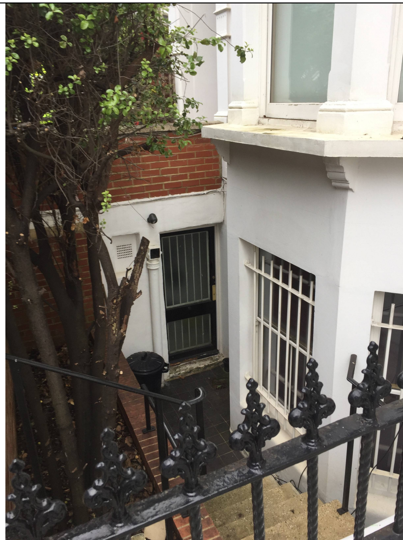
Plate 16: Adjacent property, no. 37 Pilgrim's Lane (basement).
