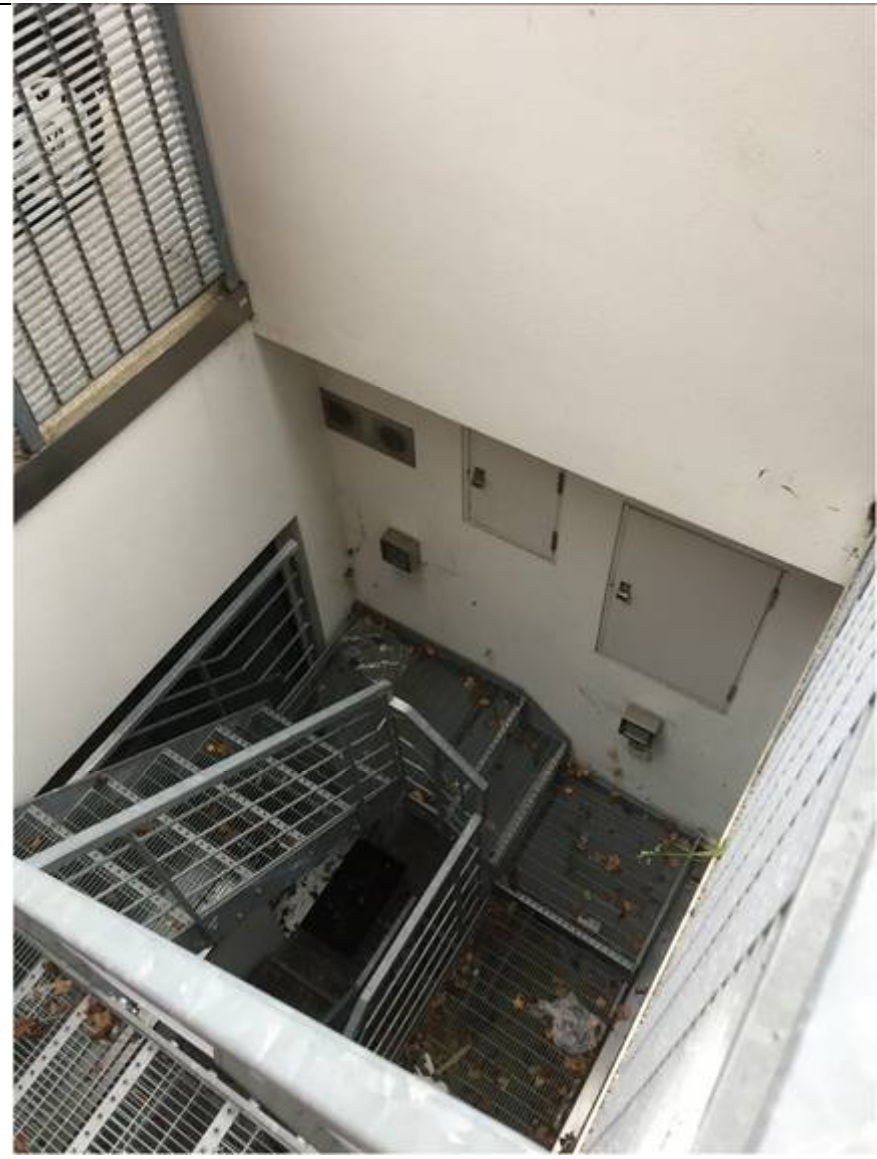
Plate 10: Adjacent property, 49 Denning Road (basement).
