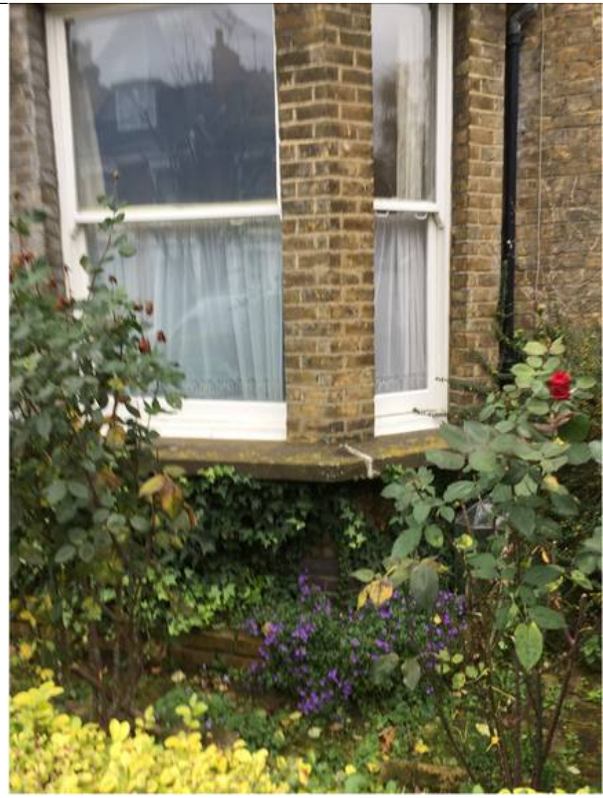
Plate 8: Neighbouring property, no. 54 Pilgrim's Lane (absence of basement).
