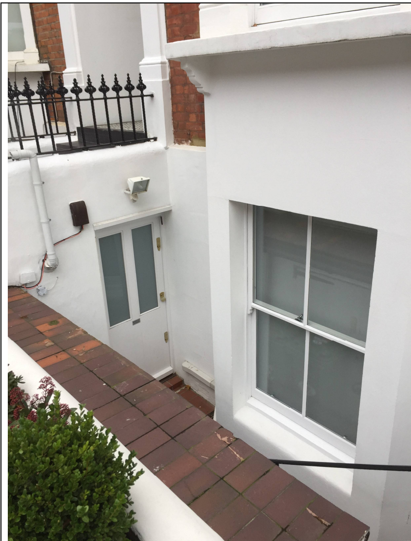
Plate 15: Adjacent property, no. 37 Pilgrim's Lane (basement).
