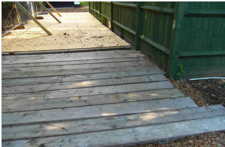
Fig.2 Side-butting scaffold boards and covered and fixed with 20mm OSB boarding
