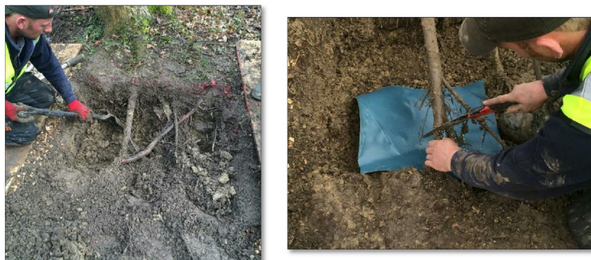
Fig. 3 Root exposure and careful pruning
