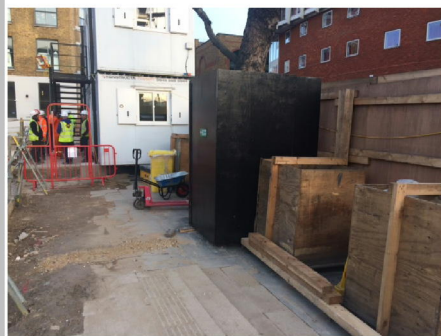
Robust hoarding and temporary concrete ground protection
