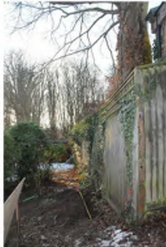
Photo 24. Trench 2 after excavation.
