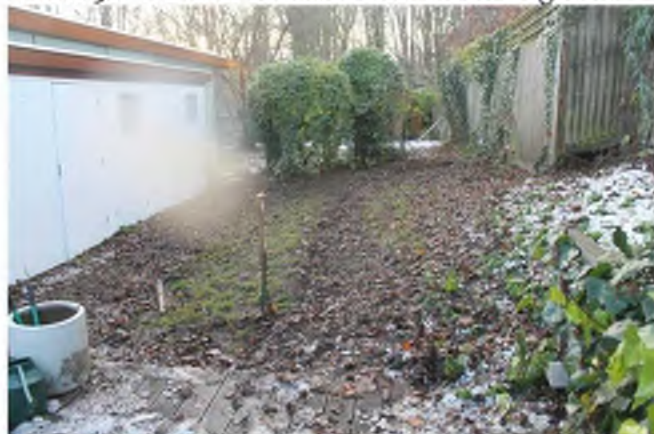
Photo 30. Trenches backfilled after the investigation.
