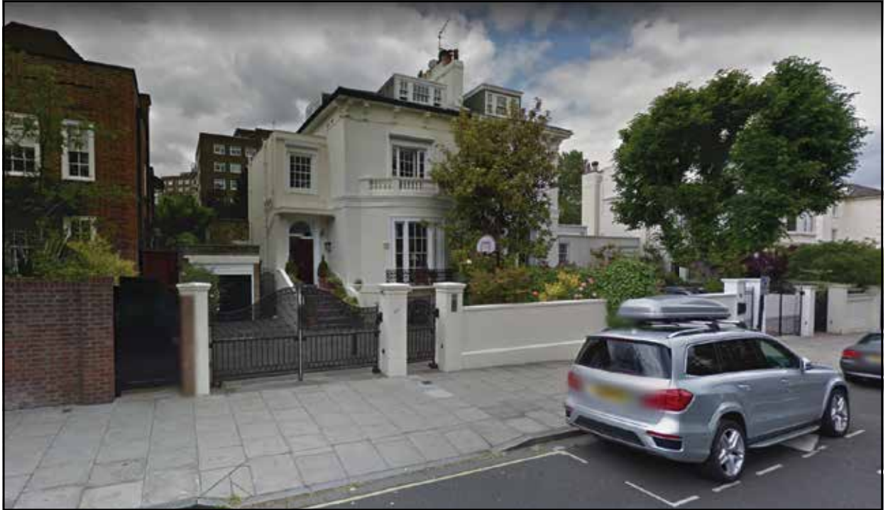
IMG-04 - Front - Existing architectural detailing to be matched
