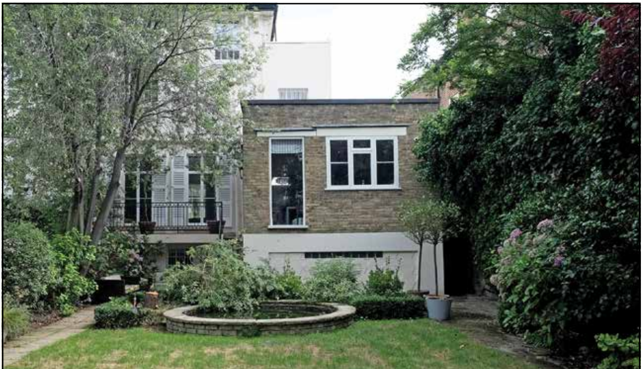
IMG-05 - Rear - Existing facing bricks to be matched where specified in proposed extension
