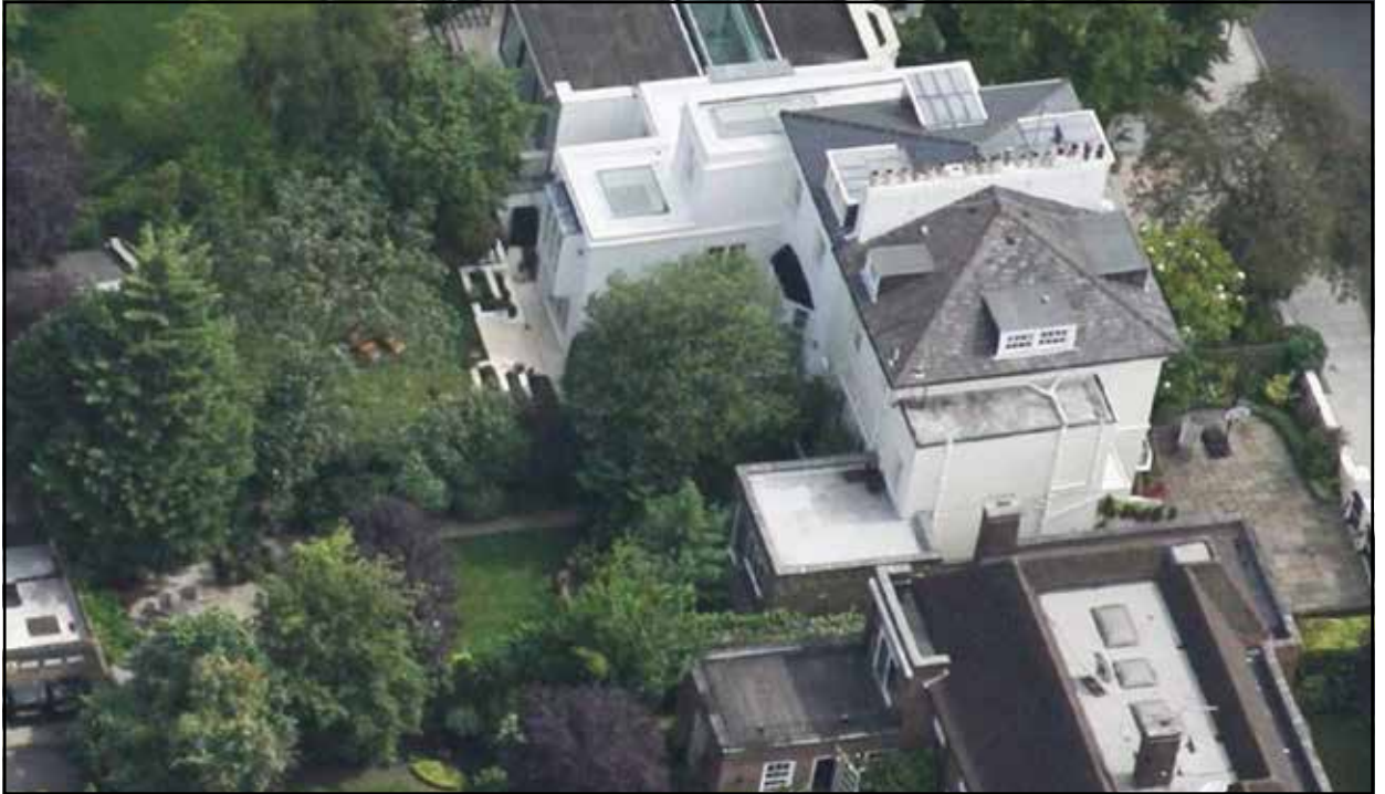
IMG-01 - Aerial - Building line established by previous neighbouring extensions
