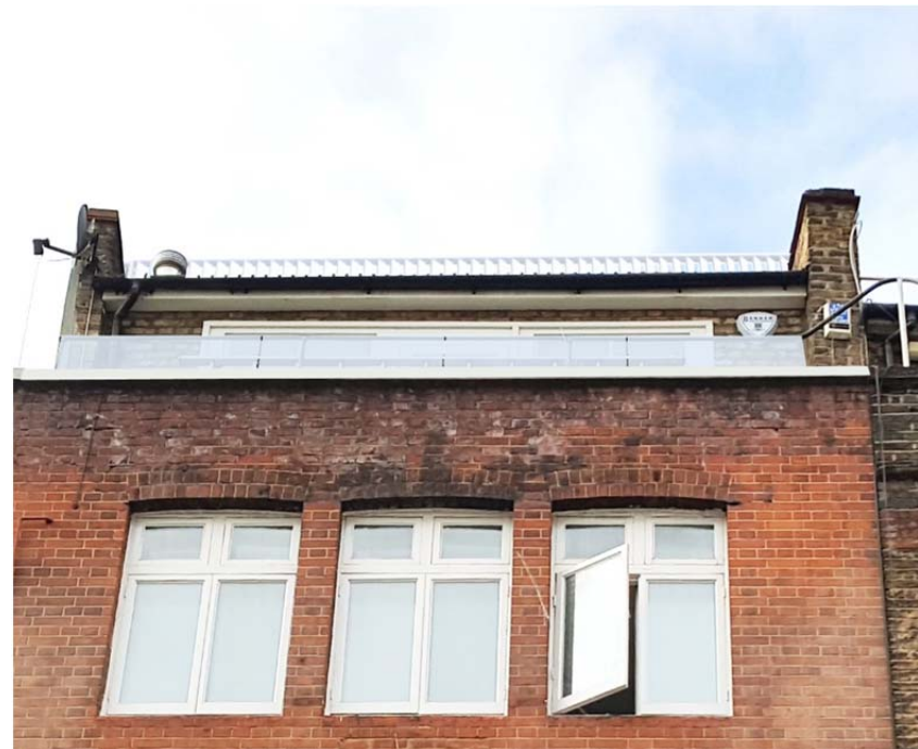
Proposed front elevation with new reduced height louvred screen, fourth floor glass balustrade and new stone coping.
