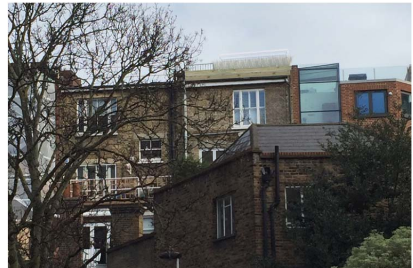
Distant view of the no.48 roof terrace, including pergola and planter
