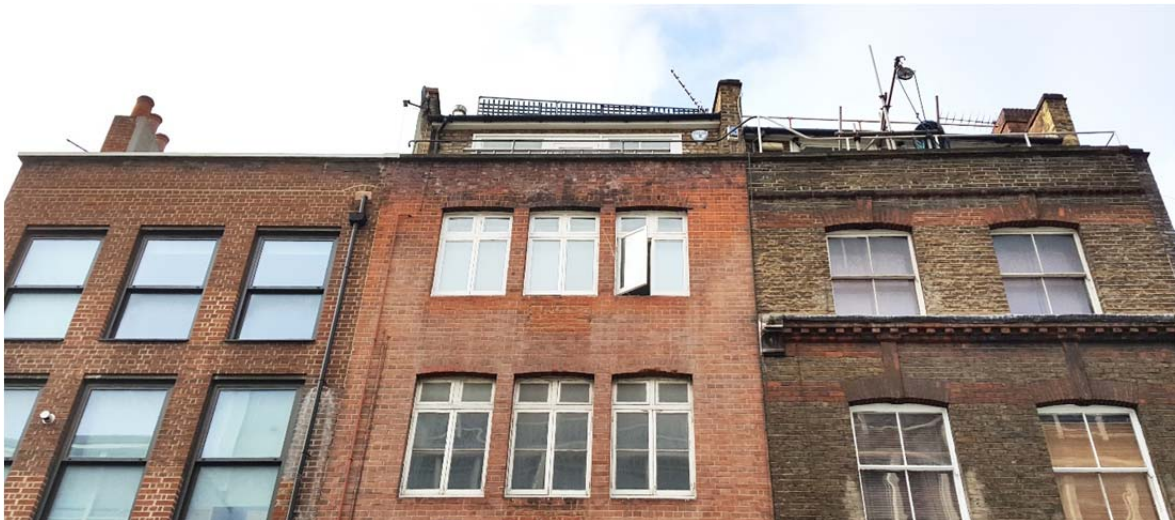
L16 | 229-001 | Planning Statement | Flat 3 rd and 4 th Floor, 48 Red Lion Street, WC1R 4PF
