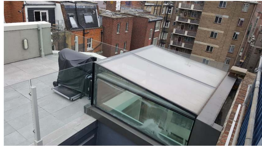
View of glazed stair boxing at no.49, and varied rear elevations to the South-West of the building.
