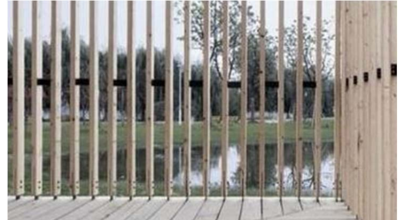
Timber louvred fencing
