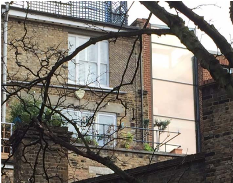
Existing view of the no.48 rear terrace from Lamb's Conduit Passage
