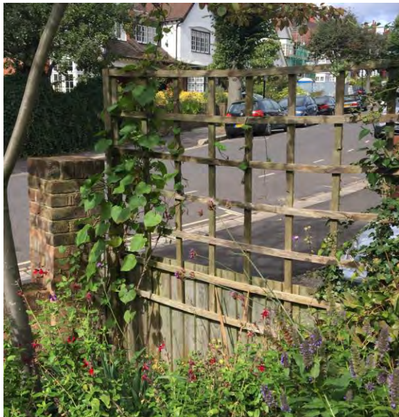
NORTHERN BOUNDARY FENCE, TO BE REPLACED WITH CLOSEBOARD FENCE TO TOP OF PILLAR WITH TRELLIS ON TOP.
