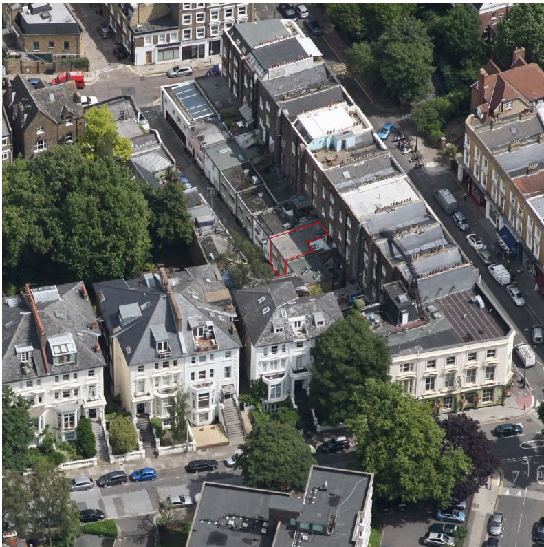
AERIAL VIEW FROM SOUTHWEST
