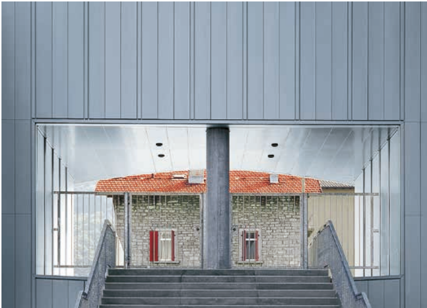
Telecom Giubiasco, Giubiasco, Switzerland
