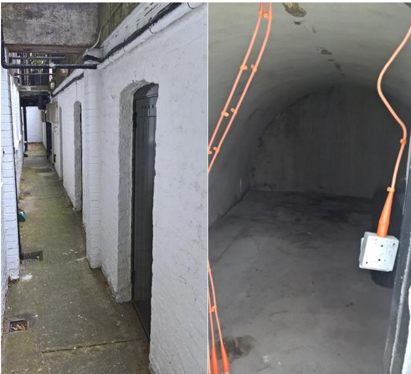
Figure 2: Lower Ground level lightwell to vaults and internal of vault 5
