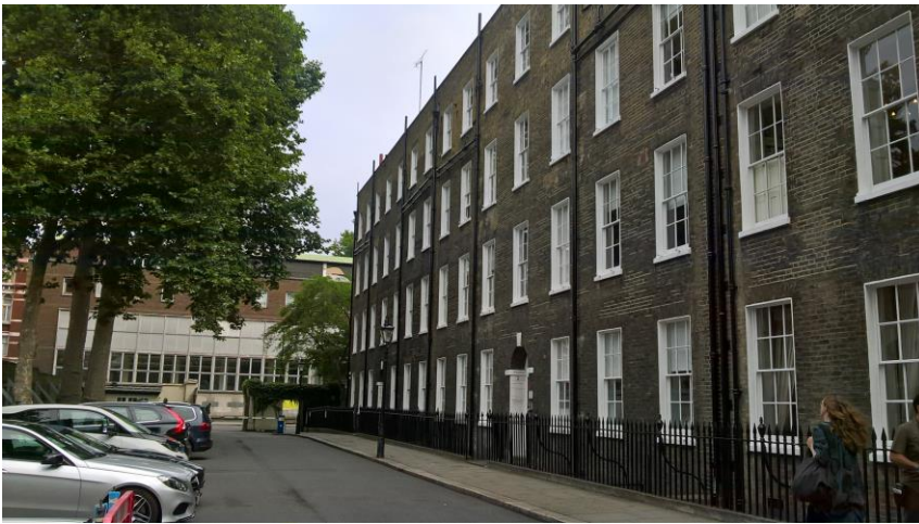
Figure 1: Front Elevation of Raymond Buildings
