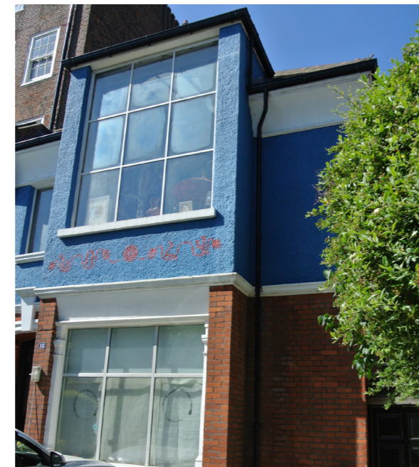
Projecting bay at no. 12 Glenilla Road
