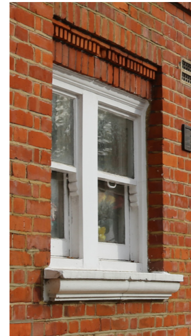
Example of deep brick reveals along Glenilla Road
