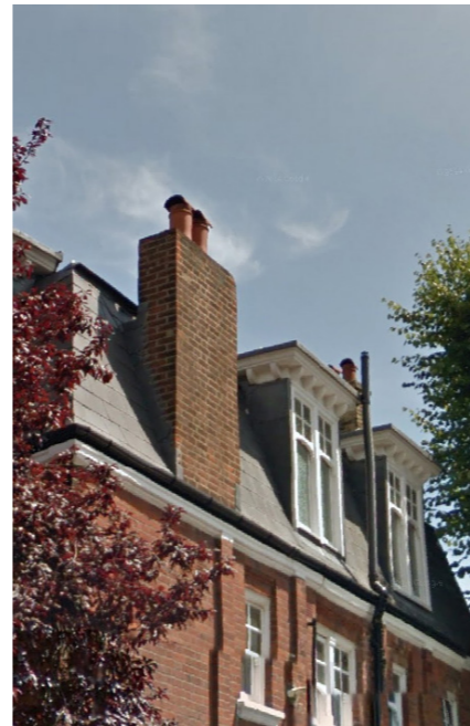
Example of a brick chimney on Glenilla Road
