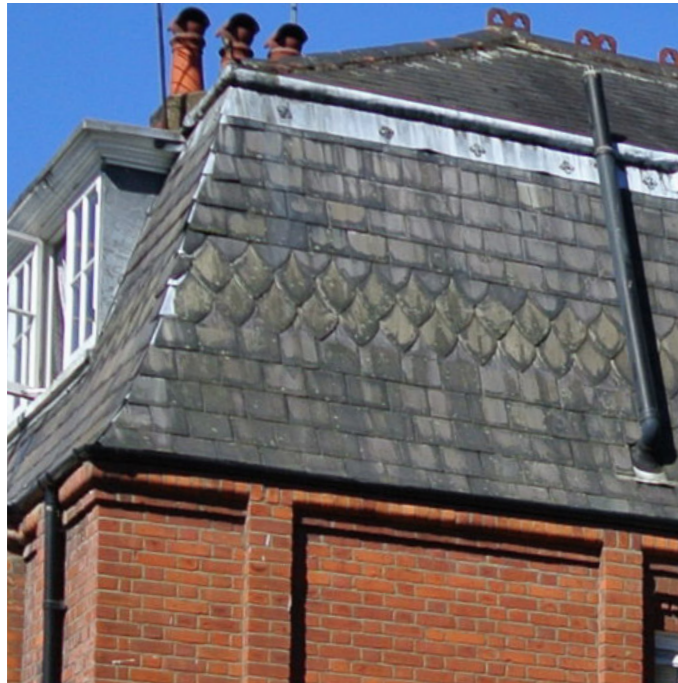
Images above - examples of local slate roofing showing a mixture of angular and scalloped tiles
