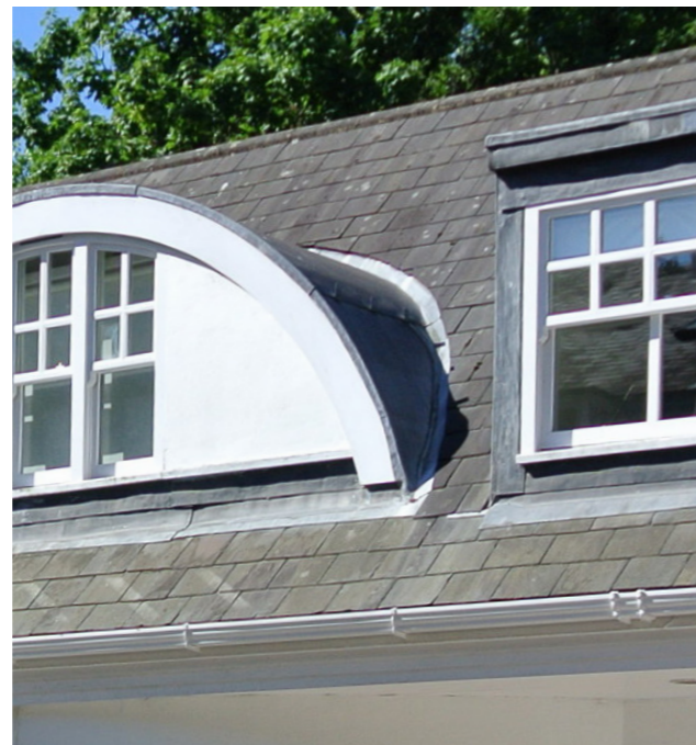
Images above - examples of local slate roofing showing a mixture of angular and scalloped tiles
