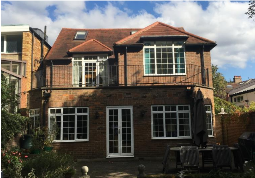
Figure 3.16 – The rear of No.30 Glenilla Road
