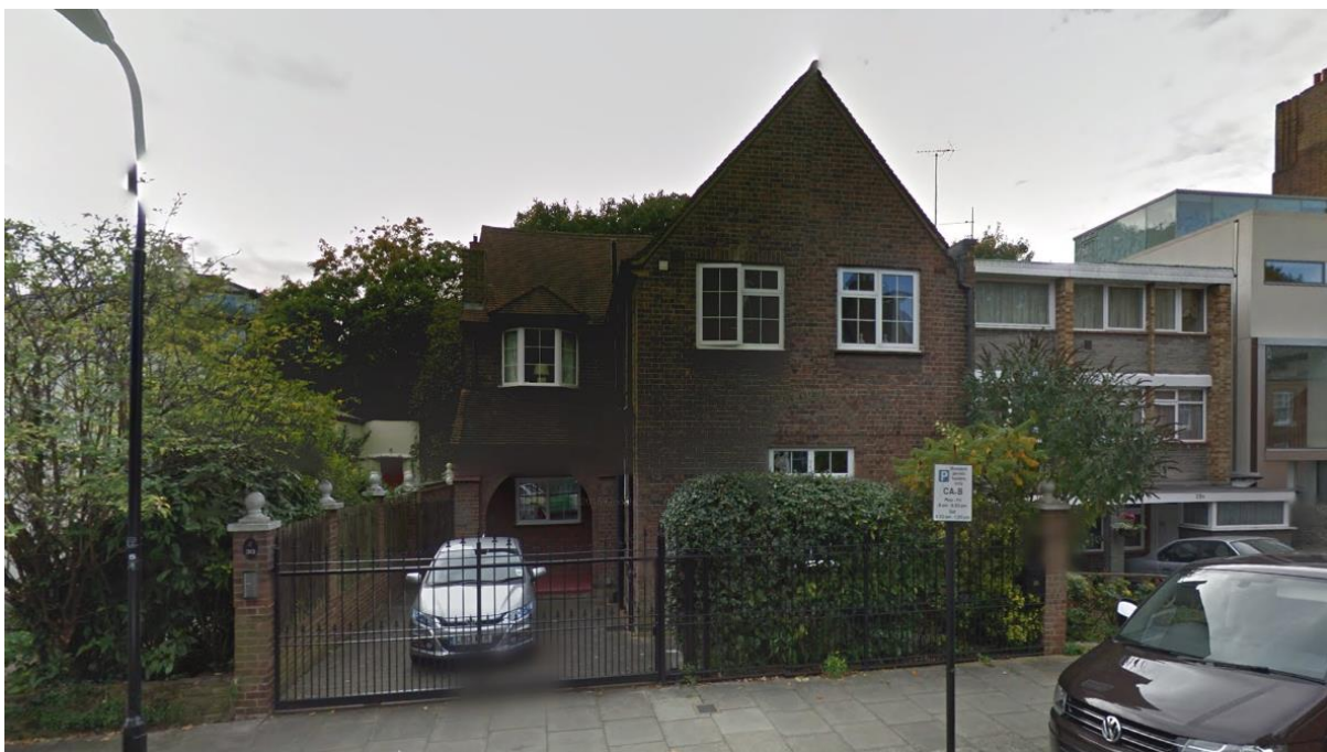
Figure 2 Existing Building (Copyright © 2017 Google)
