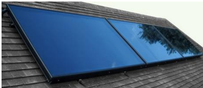
Figure 11: Example solar thermal “flat plate” collector
