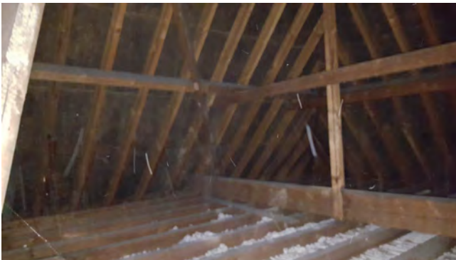
Northeastern eaves space
