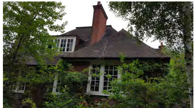
View of rear façade from garden
