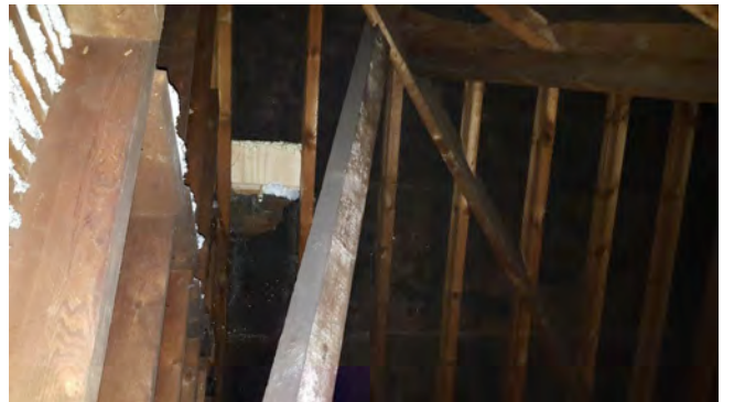
Opening in northeastern eaves space
