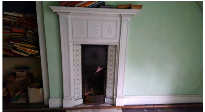
Blocked up fireplace
