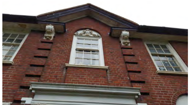
View of front façade of the house
