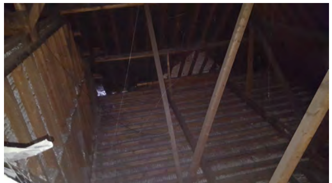
Opening in the loft space
