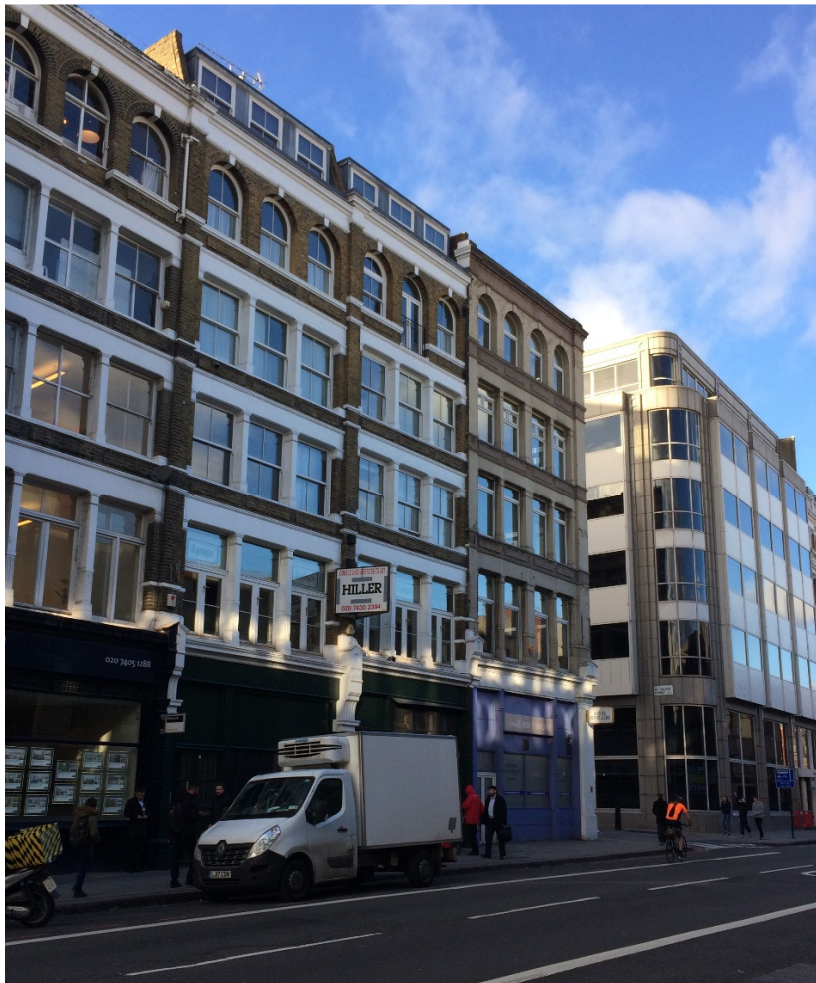
The building as existing viewed from Farringdon Road, looking north
