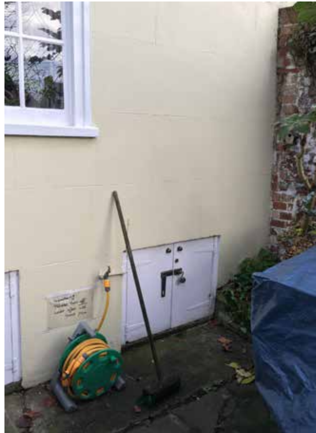
Figure 6. Existing timber doors to undercroft storage.
