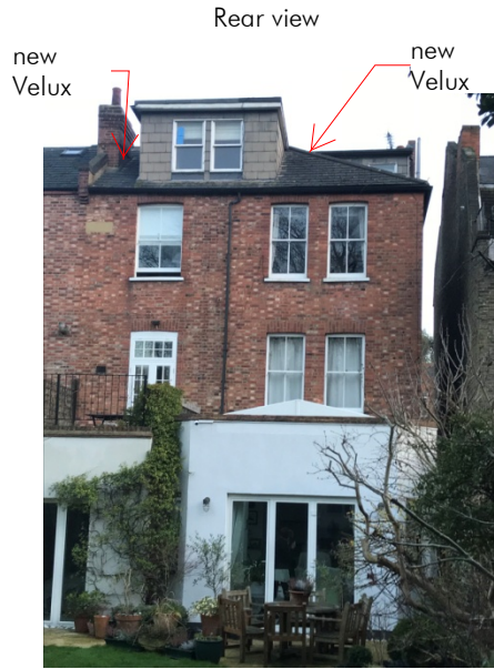
Section of roof area facing west
