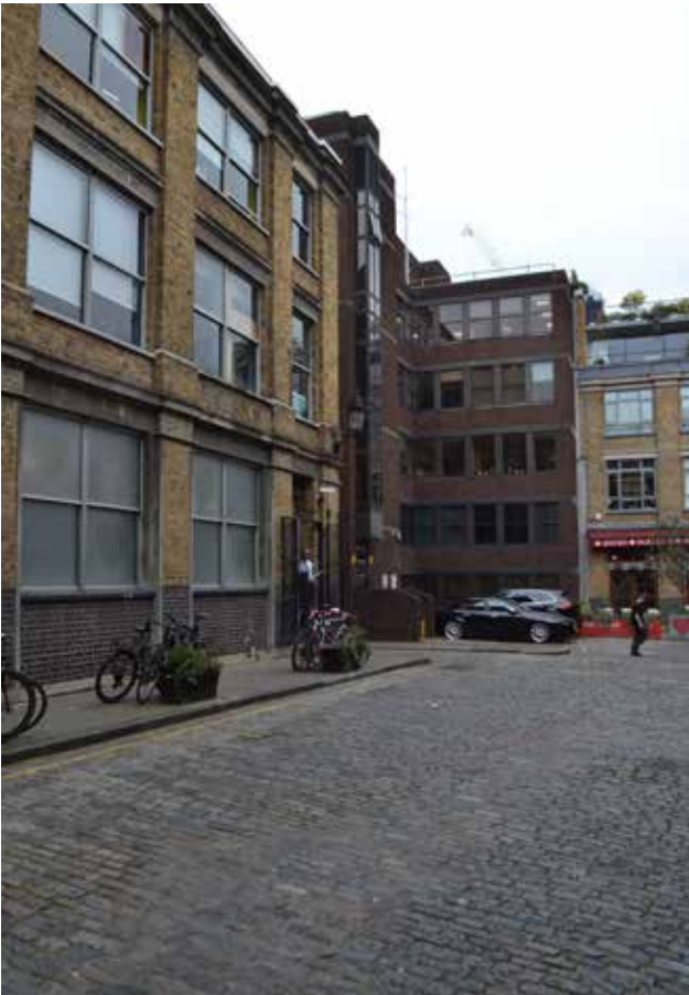
49. Rear elevation of No.20-23 Greville Street
