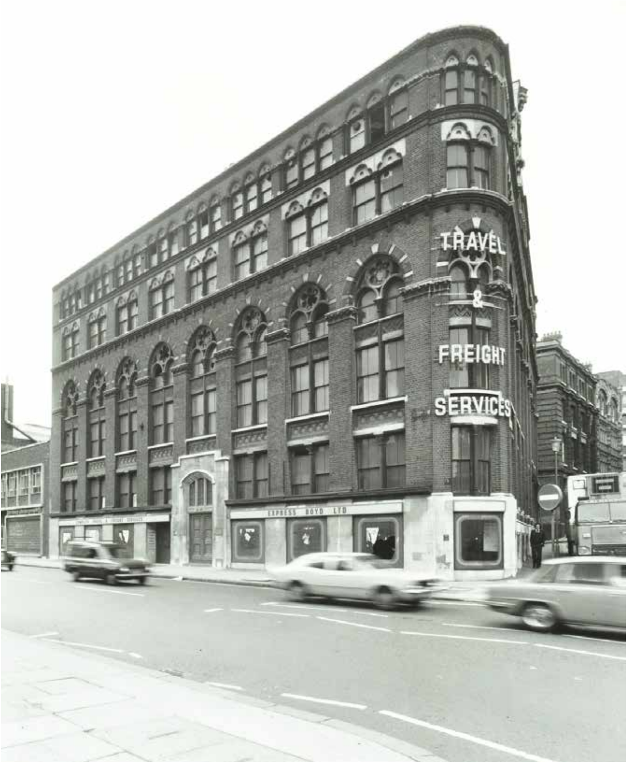
30. Photograph showing view from Farringdon Road looking towards Greville Street, 1977, Collage
