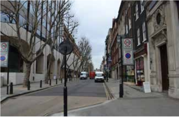
38. Hatton Garden, looking north
