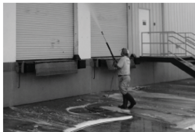
Fig. 105. External Cleaning – Pressure washing the outside
