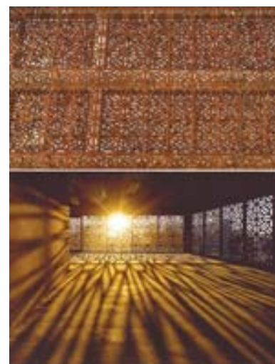
Fig. 133. Bronze roof perforated terrace covering.
