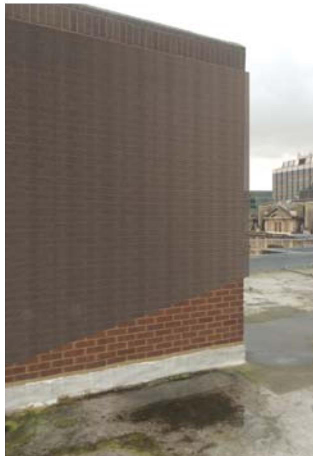
Fig. 85. Mesh test panel shown over existing brick wall.
