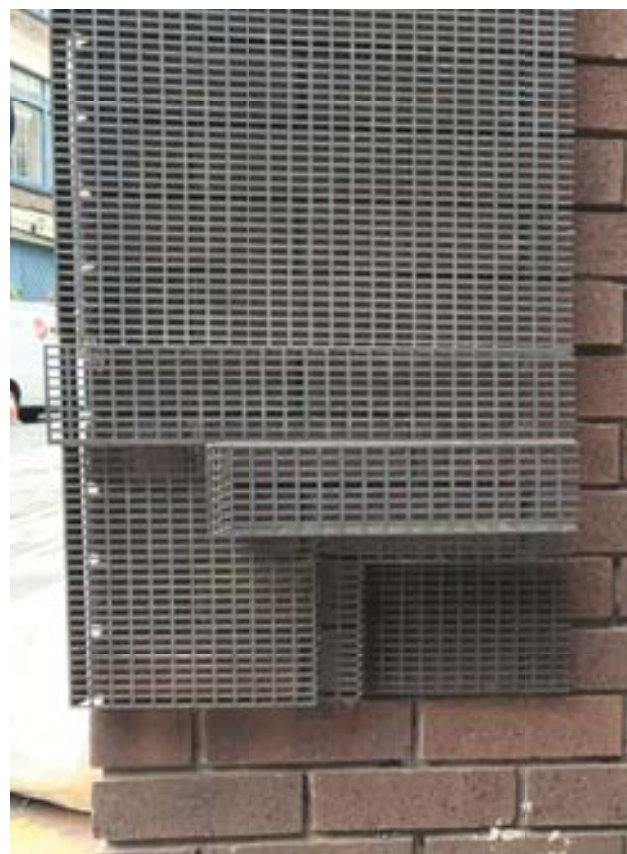
Fig. 88. Previous mesh test panel shown over existing brick wall. This is a test sample only and does not represent the finish/pattern of the proposed facade material.
