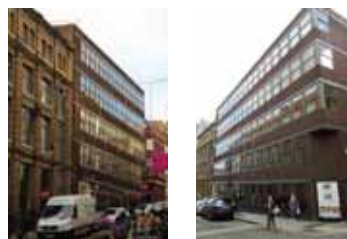
Existing building at 20-23 Greville Street.
