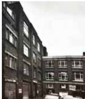
Photograph showing rear elevation of 20-23 Greville Street.
