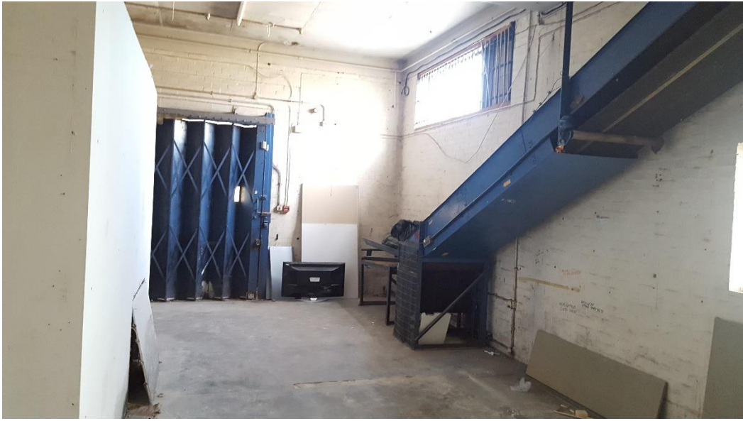
Image 7 – Service door and conveyor belt
