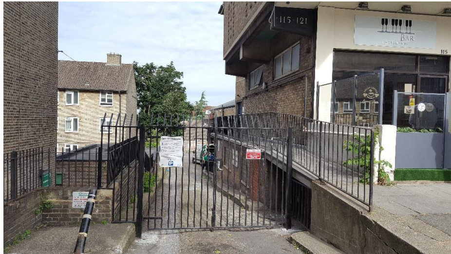
Image 1 – Entrance to the site from Finchley Road
