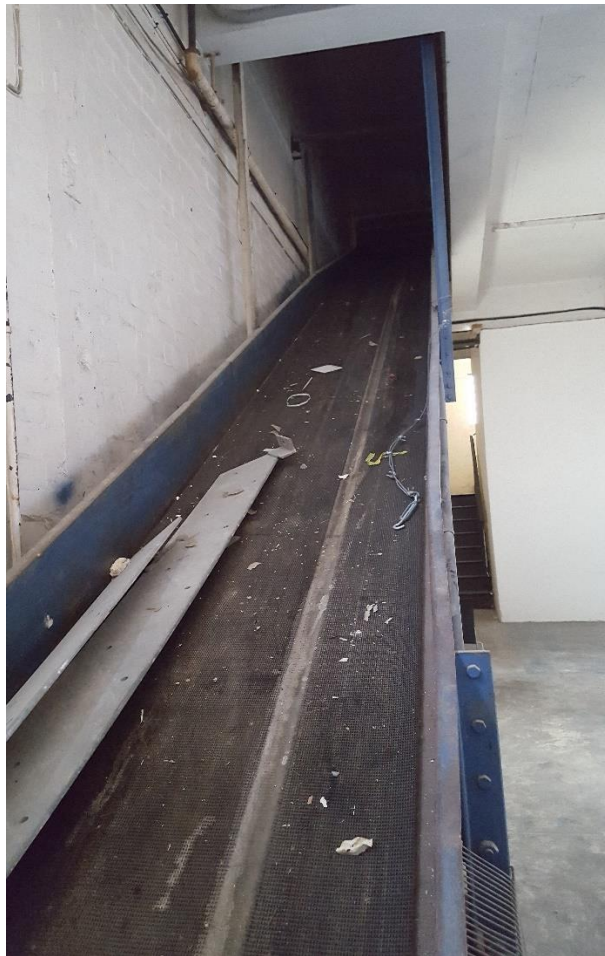
Image 8 – Conveyor belt to upper ground floor level
