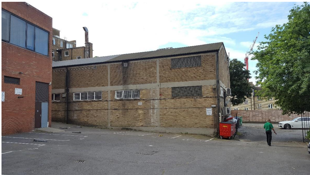
Image 6 – Image of unit from car park off Belsize Road
