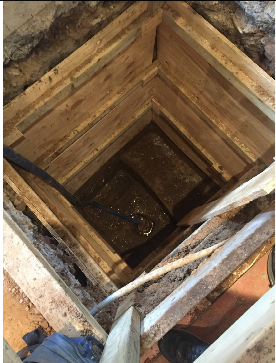
Plate 2: Trial pit following pumping out of groundwater.
