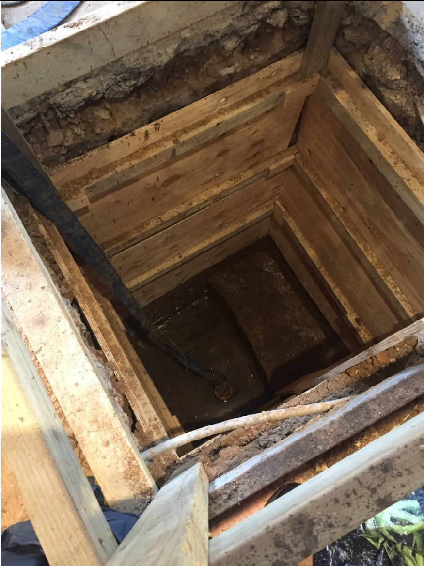
Plate 1: Trial Pit with groundwater visible.
