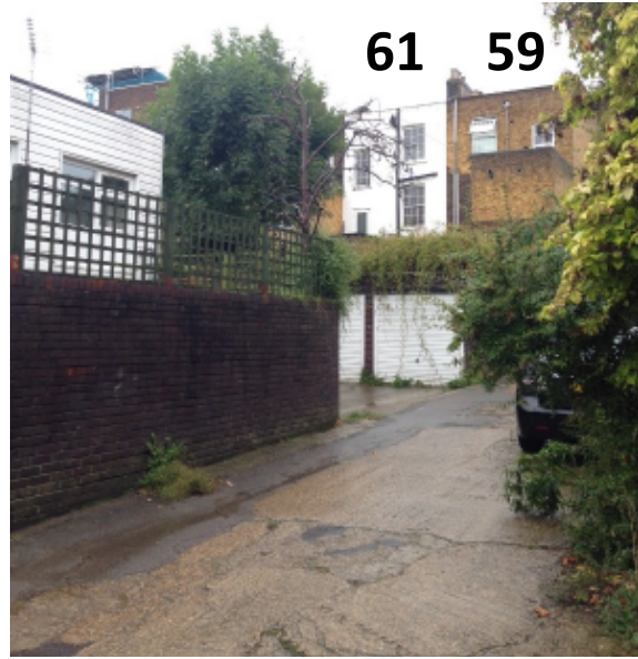
2) Rear elevation of application site and no.59, taken from Torriano Cottages
