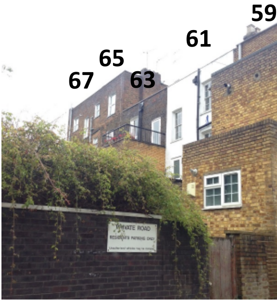
1) Rear elevation showing existing extension and terrace at no.63, and extension in similar style at no.59
