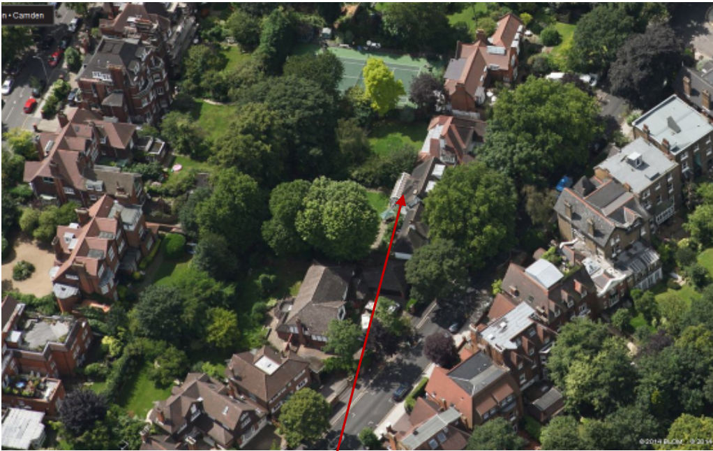
1. Aerial photo of the site showing the site before demolition commenced
