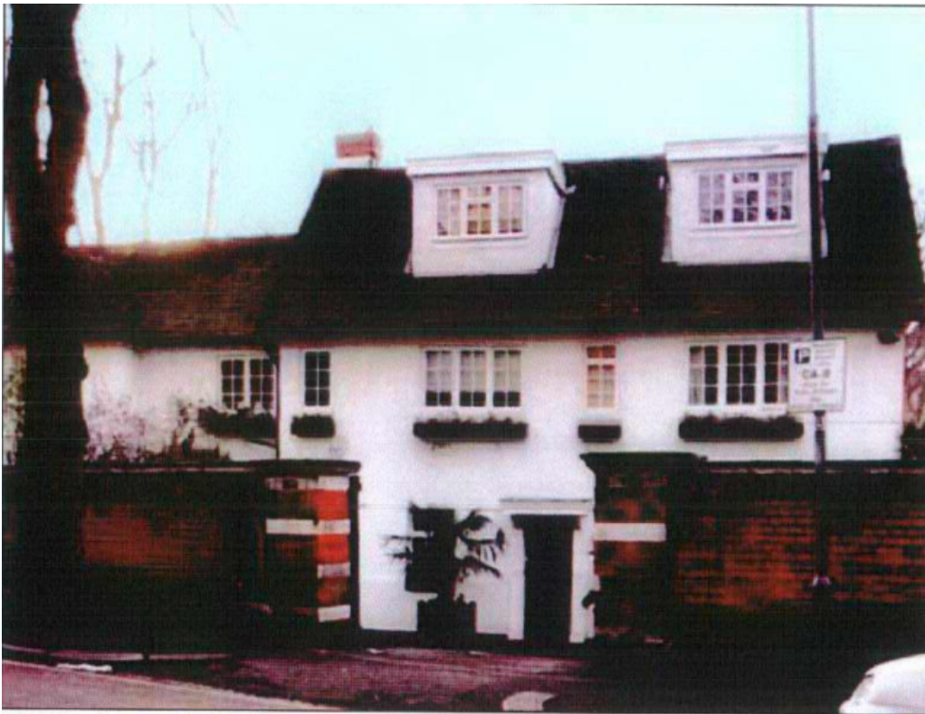
2. Archive photo of pre-existing house
