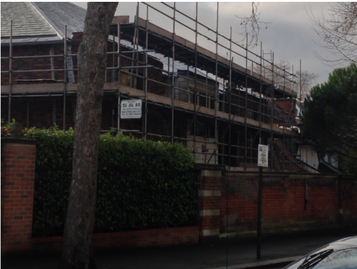
4. View toward partially completed house (hips and pediment still to be constructed)
