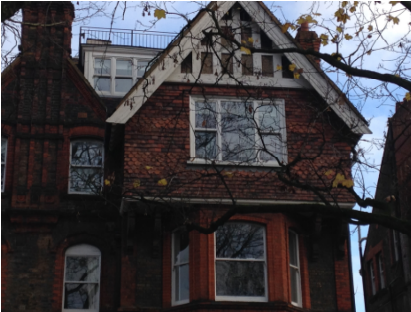
5. View toward property in adjoining road (Strathray Gardens) showing triptych window consisting of fixed pane of glass and 2 sash windows either side
