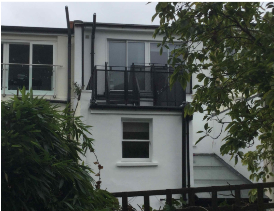
Photograph 2. Existing rear dormer doors/balustrade.
