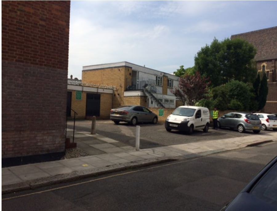
View of the appeal property from the south-east with the church of St Silas The Martyr in the background
