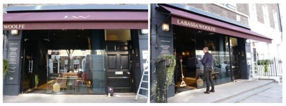
The existing shop front, installed in 2008, is fully glazed with minimal fixings. The panelled timber door and square fanlight on the right hand side have not been altered. We propose that the existing fully glazed shop front is replaced with a combination of glazing and timber panelling, to reflect both the property's historic character and local guidance regarding shopfront design (please see next page).
