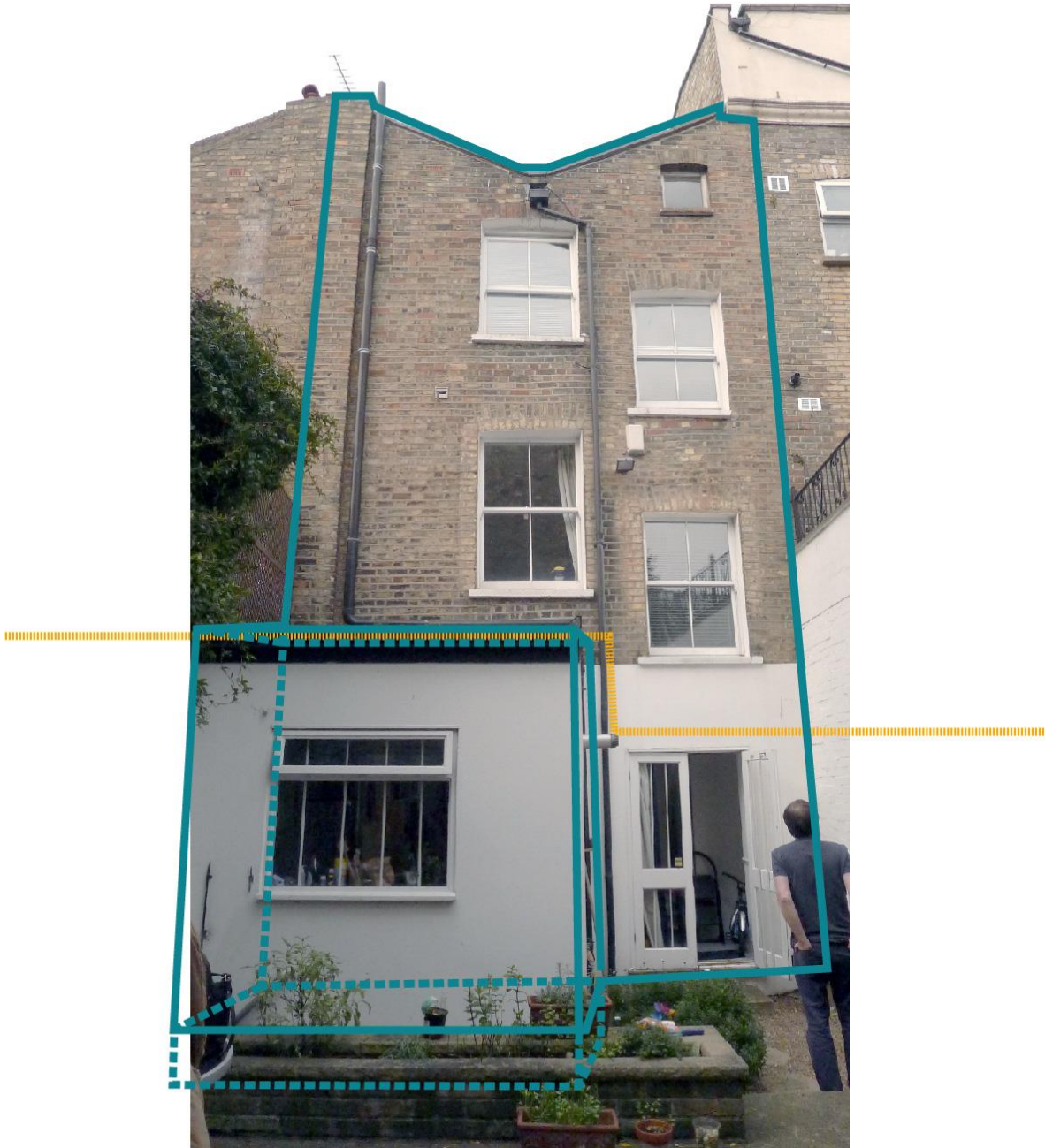
134 Torriano Avenue, existing rear elevation
