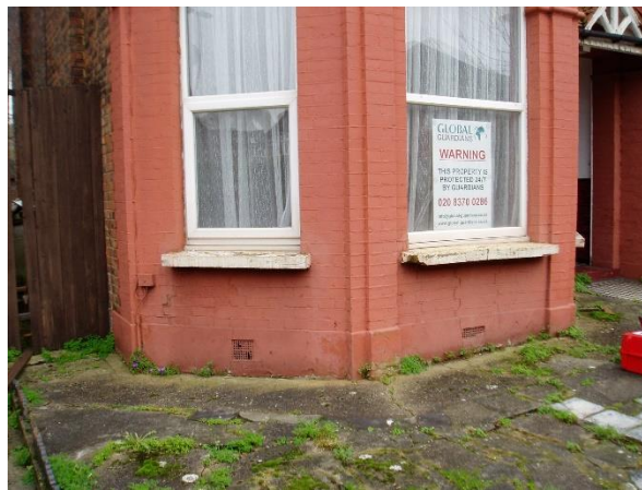
Fig. 2. Front yard with extensive hardstanding
