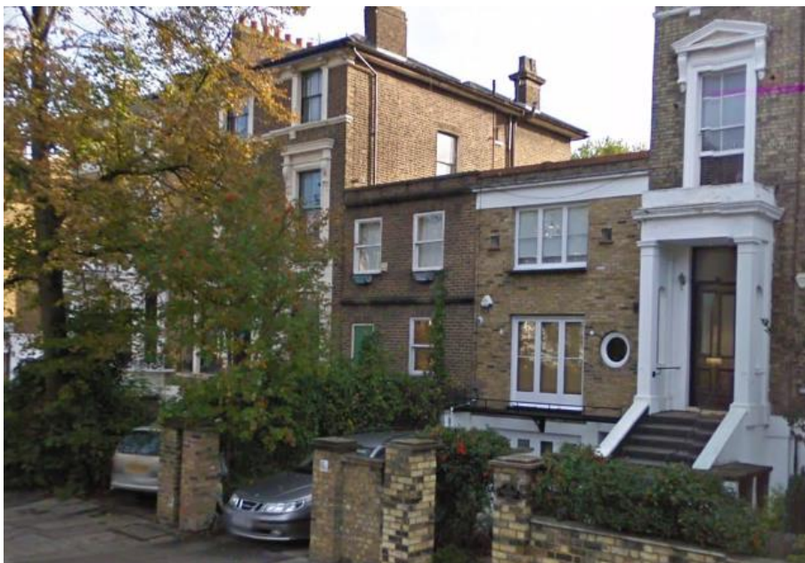
Figure 1: Existing building (centre), view from Parkhill Road
