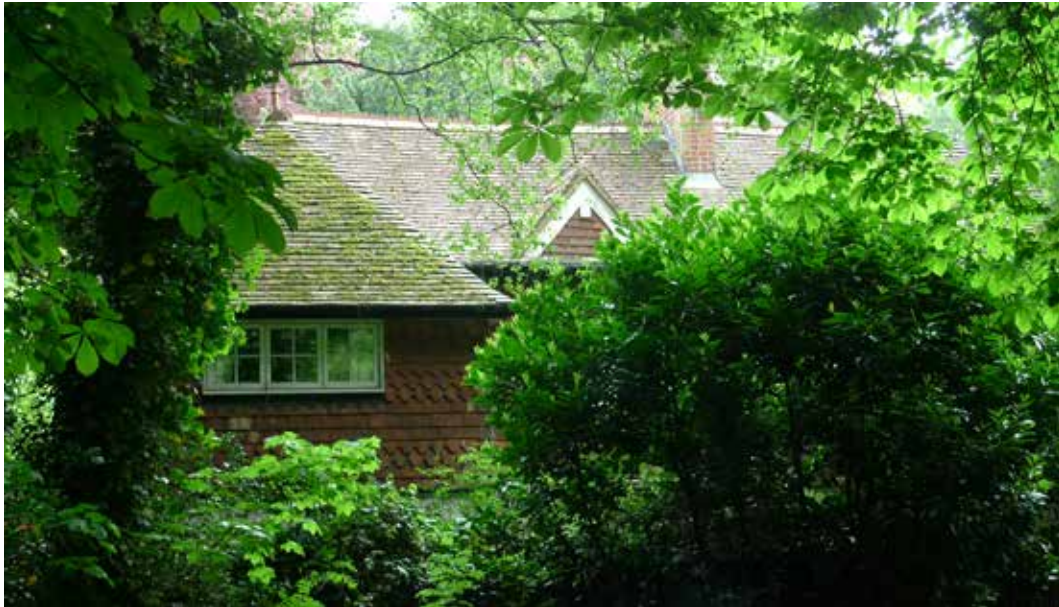
West facade seen from North End Road (May 2017)
