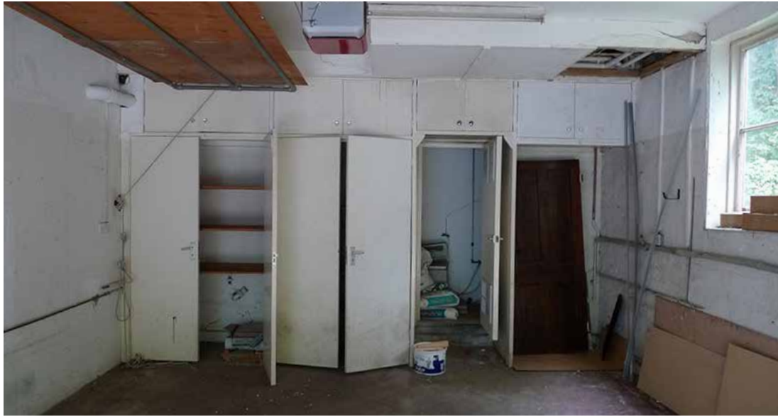
Garage interior, off of internal courtyard
