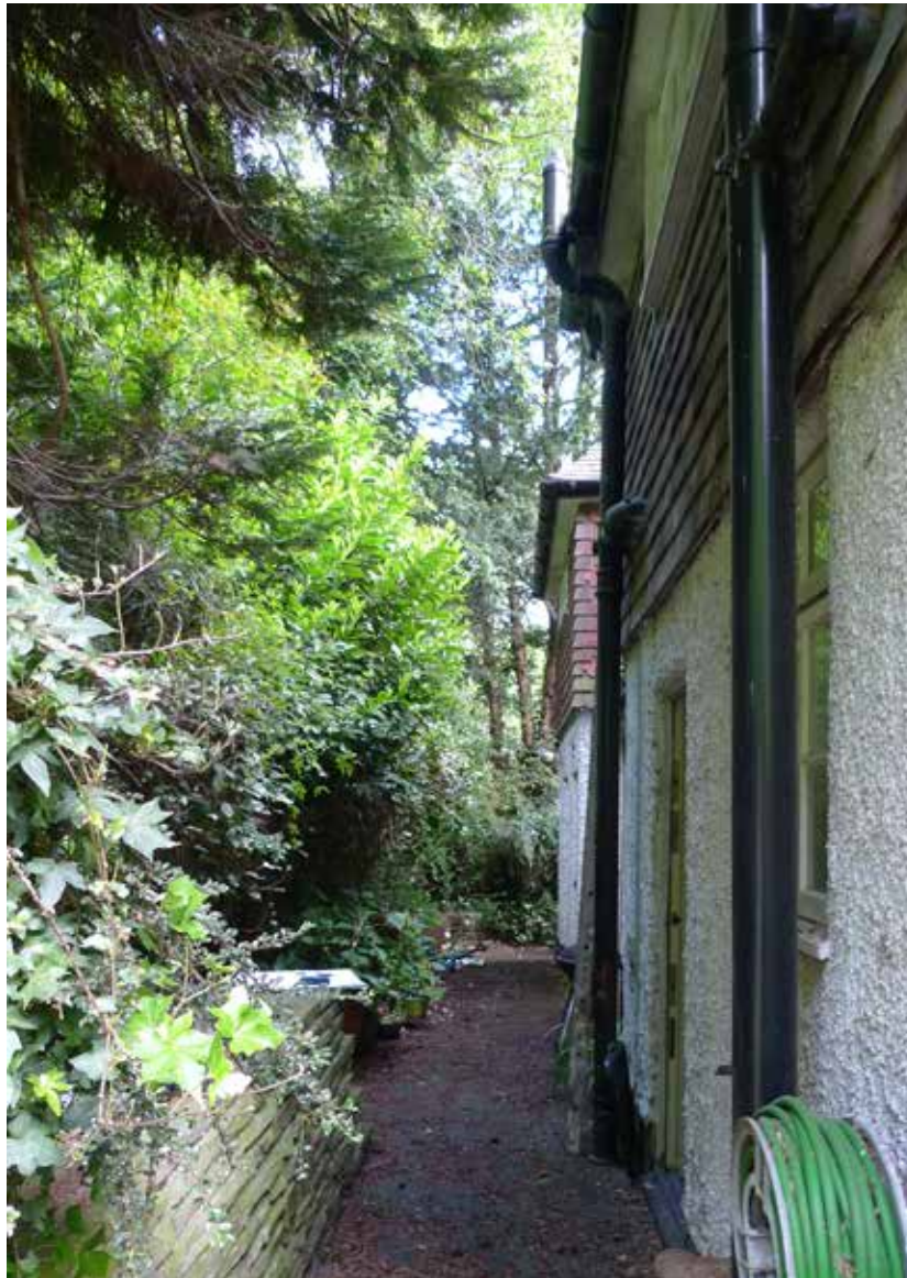
Access along west facade (May 2017)
