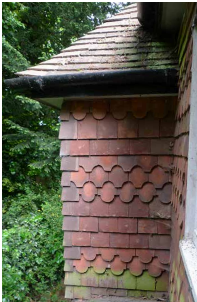
Terracotta tiles lining upper storey external walls
