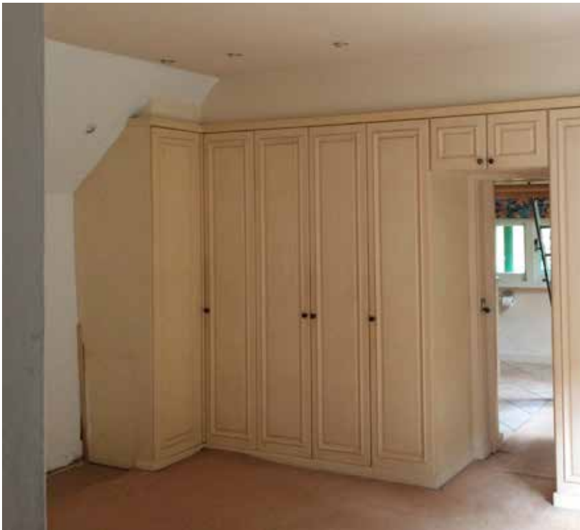
Interior of west wing with lowered ceiling and fixed wardrobes.
