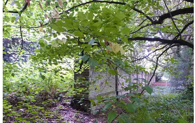
Directly to the west of The Lodge lies 18th Century boundary wall of Pitt House, demolished in 1954. Brick wall, no return, approximately 2.4m high running 30m until Terrace House, pillasters every 3m.
