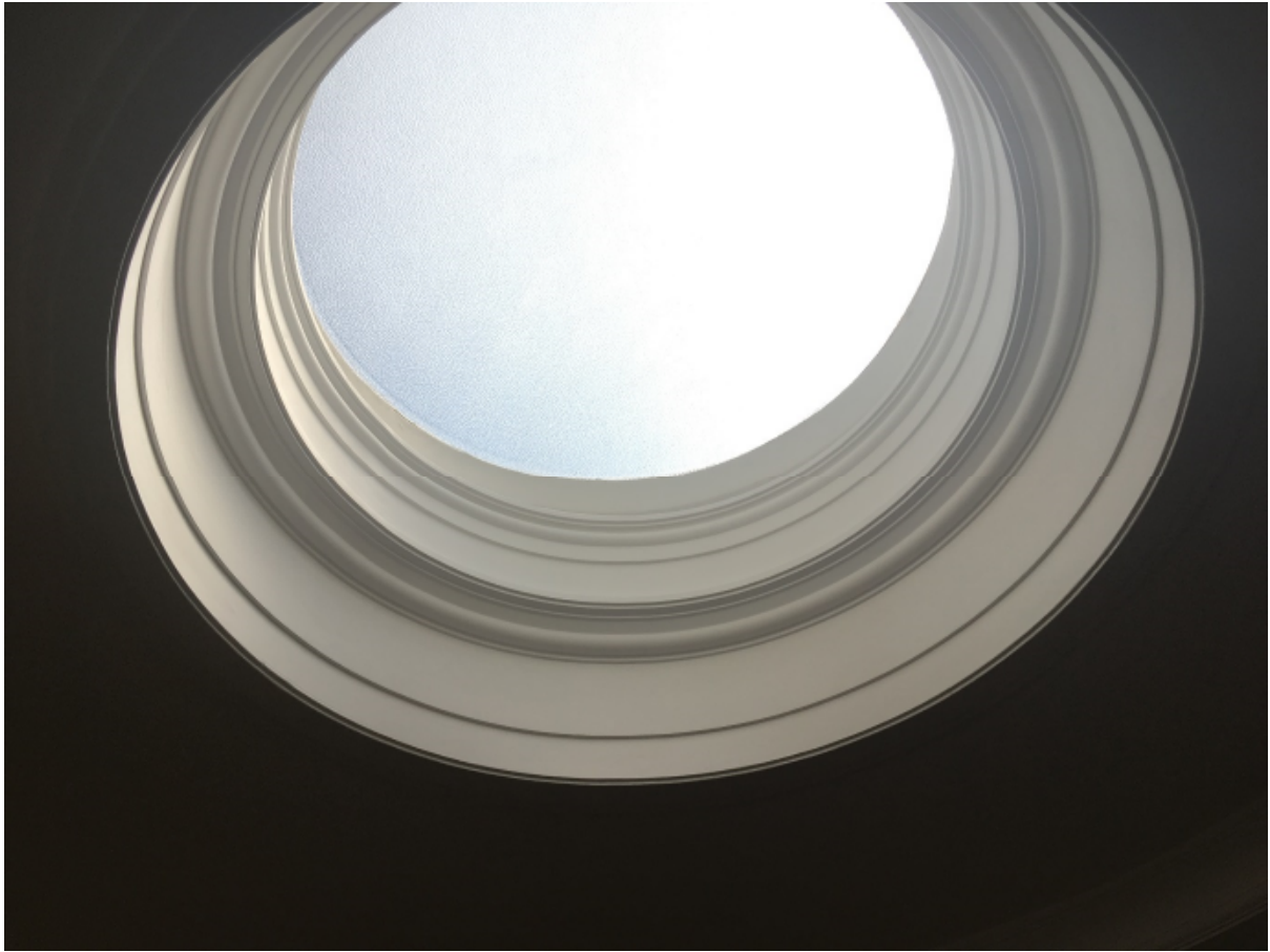
Rooflight in attic floor
