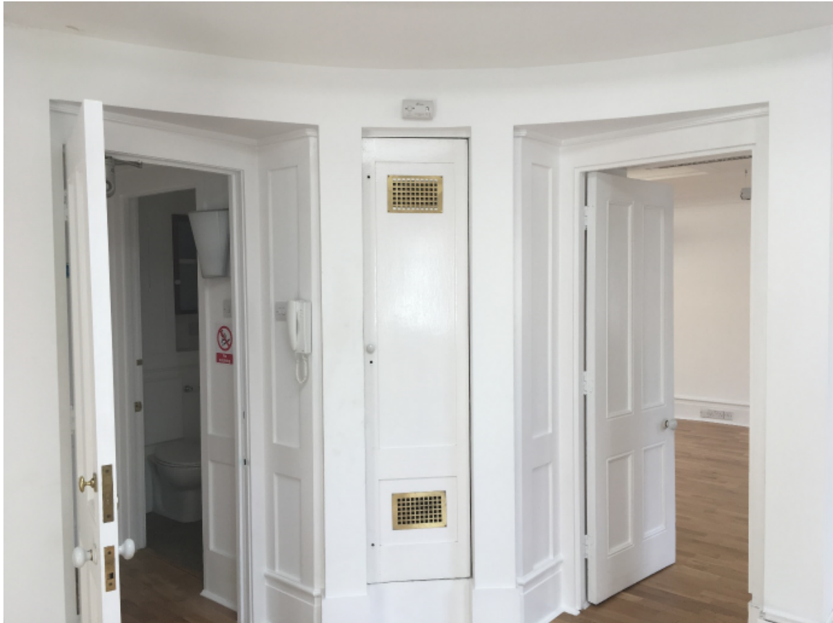
Example of interior – door to right where existing opening in party wall has been formed
