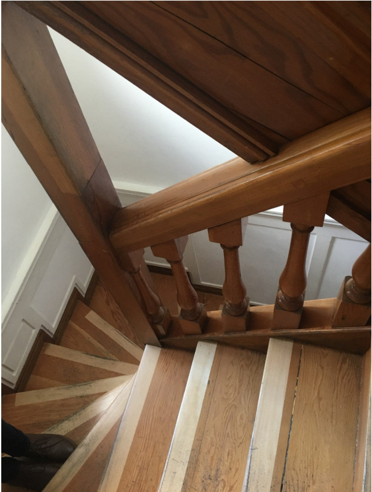
Rear Access stair to upper levels
