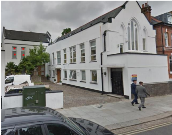
1. Trinity Close photograph taken from Willoughby Road - red dots denote living area windows of no.1
