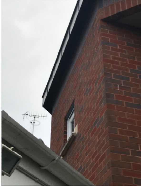
4- 5 Rear elevation and subject window (above rear conservatory extension)
