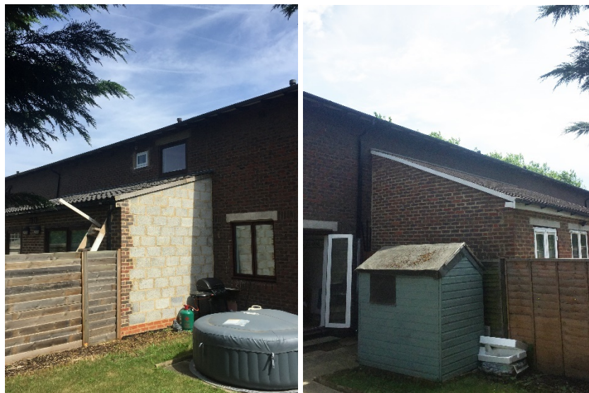
Extensions to the rears of no. 62 and 60 Westcroft Close, left and right respectively.
